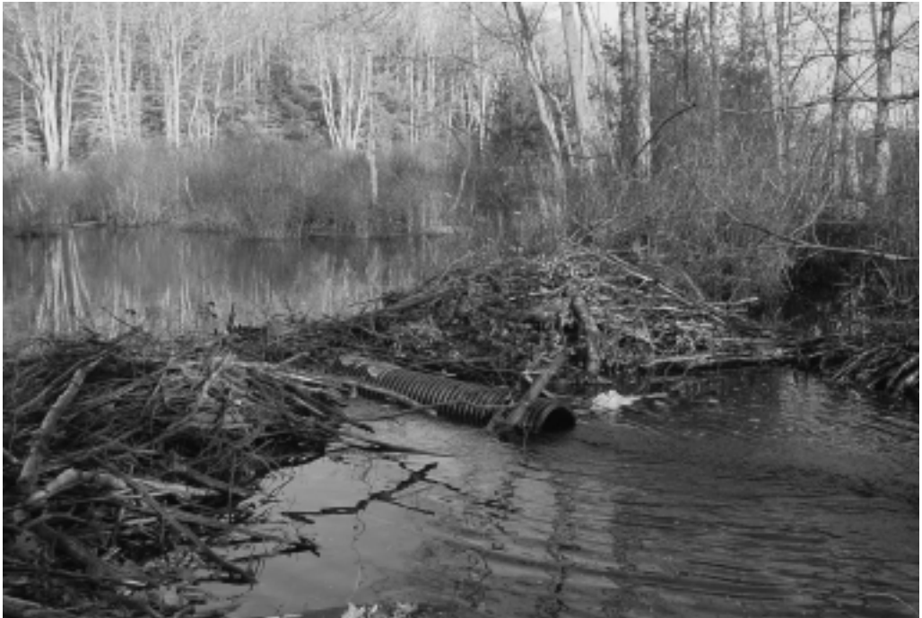
Photo 2. A Castor Master™ with a submerged polyethylene pipe 0.3 x 12 m. If pipes are placed so there is little difference between the water level above and below beaver dams, fish can easily swim through. Photograph: David Wilkins.
