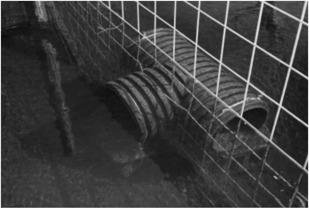
Photo 4. A 30 cm polyethylene T-joint in the front of this Beaver Deceiver™ keeps beavers and large turtles out of traffic by allowing them to travel through the fence and therefore the road culvert. The 90° angle prohibits beavers from transferring woody damming material inside. Photograph: Skip Lisle.
