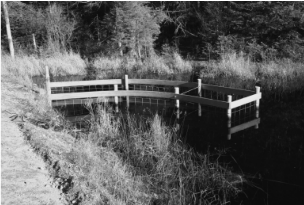
Photo 3. At narrow sites Beaver Deceivers™ should create a salient down the middle of the stream that allows beavers to swim by the front of the fence. If the fence blocks the channel, the front is likely to become a beaver dam. Crescent-shaped models like this one (perimeter: 11 m) work well at sites where the stream enters the outlet at an angle. Photograph: Skip Lisle.
