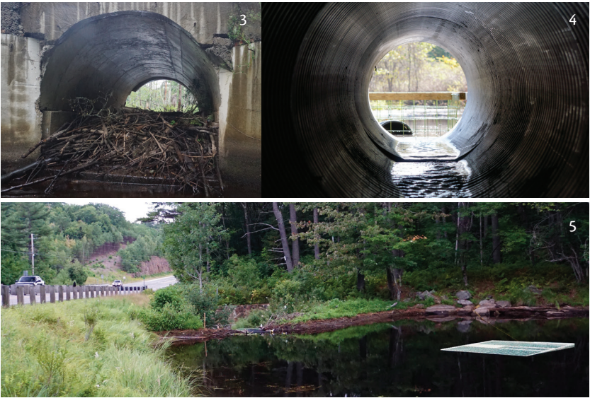
3) A common site—a beaver dam inside an unprotected culvert. 4) A previously dammed culvert now protected by a BD. 5) A beaver dam controlled, and Route 9 (north of Keene, NH) protected, by a Castor Master™ pipe system. The filter (beavers out, water in) on the end of the pipe is called a Square Fence™.
