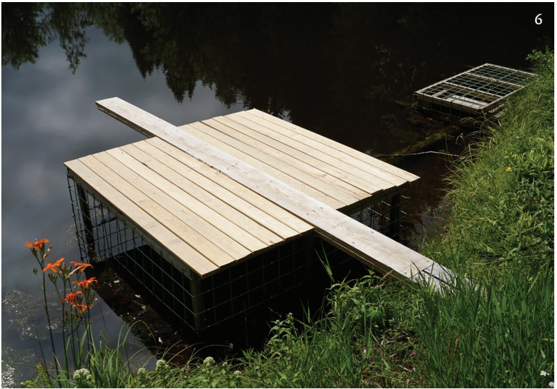
6) A Beaver Deceiver™ protecting a standpipe on a deep, steep-banked pond. It is covered with a deck and diving board.
