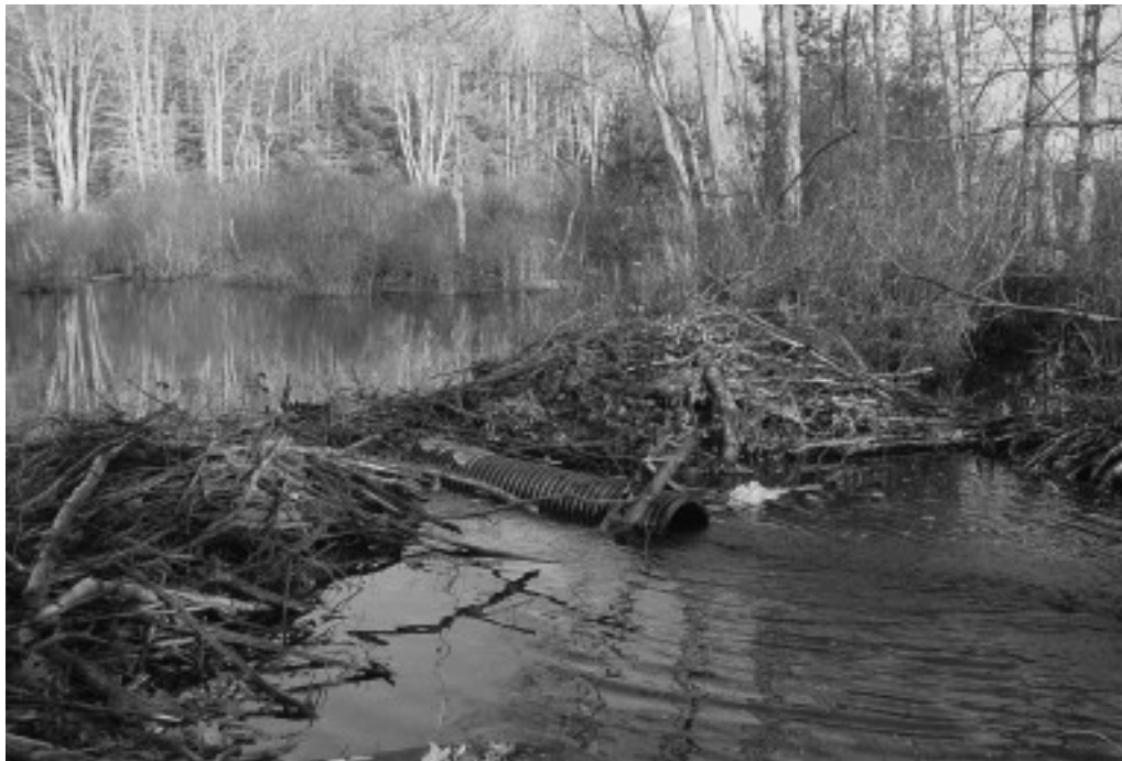
Photo 2. A Castor Master™ with a submerged polyethylene pipe 0.3 x 12 m. If pipes are placed so there is little difference between the water level above and below beaver dams, fish can easily swim through. Photograph: David Wilkins.
