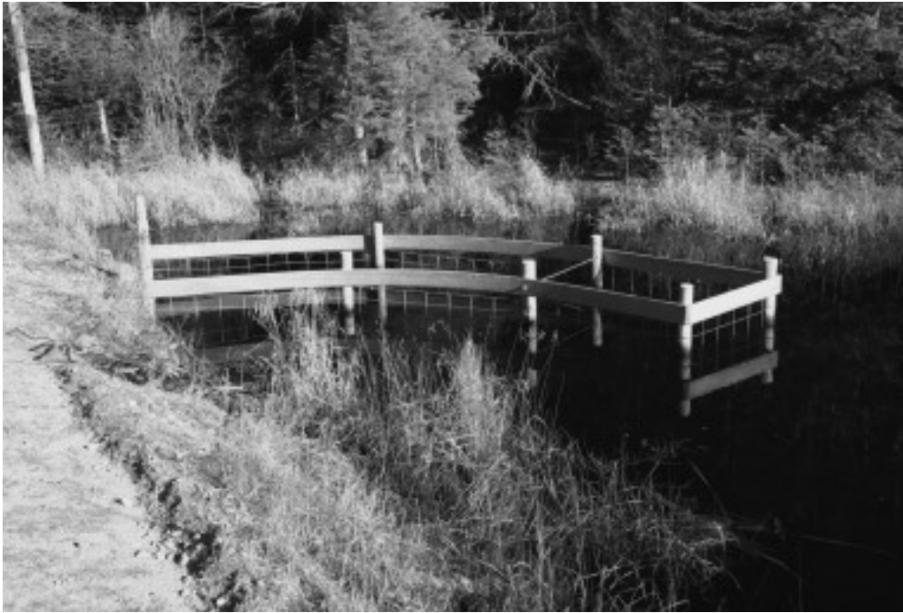
Photo 3. At narrow sites Beaver Deceivers™ should create a salient down the middle of the stream that allows beavers to swim by the front of the fence. If the fence blocks the channel, the front is likely to become a beaver dam. Crescent-shaped models like this one (perimeter: 11 m) work well at sites where the stream enters the outlet at an angle. Photograph: Skip Lisle.
