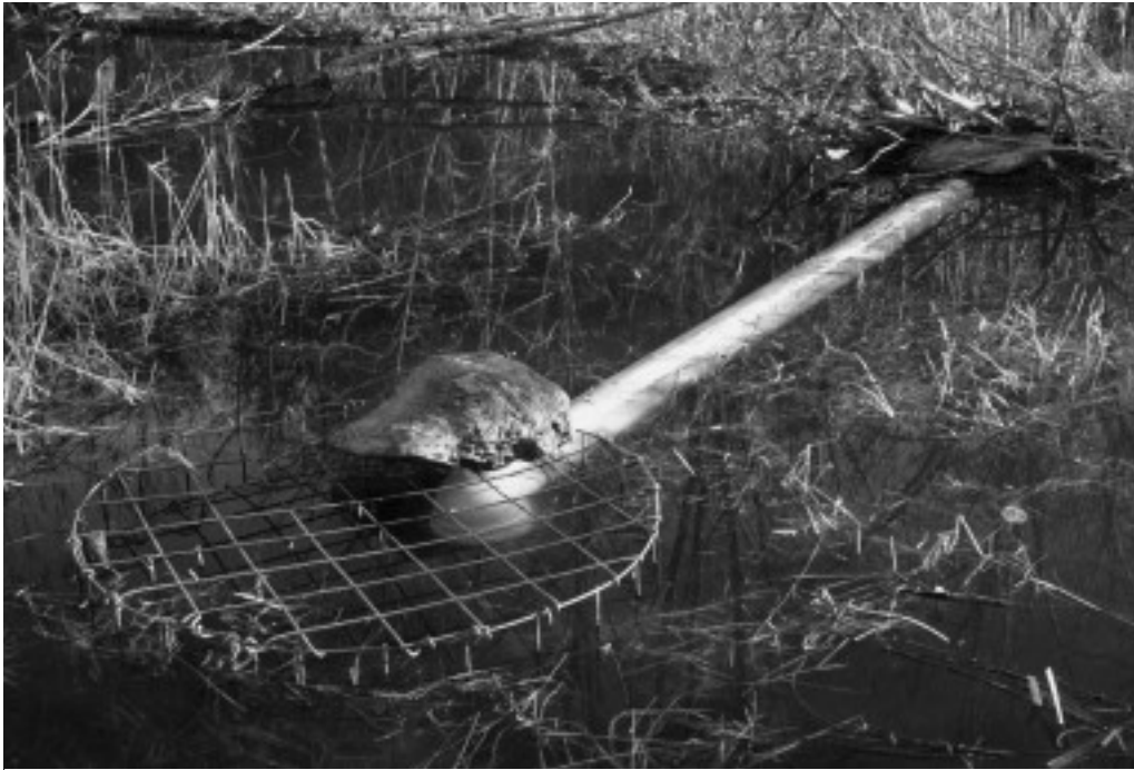
Photo 1. Castor Master™ pipe systems use a Round Fence™ (RF) for a filter. Many types and sizes of pipes can be used; this one is of polyvinylchloride and measures 0.2 x 4 m. Because the pipe is placed level it has a silencing elbow to prevent the sound of running water from escaping and attracting beavers. This RF is small (diameter: 1.2 m) and lightweight so it has a rock on top of it to help counter liquid-displacement forces acting on the pipe. The pipe is also weighted down where it ends in the dam and covered with branches so beavers cannot access it. This is a relatively small system to match a small stream. Photograph: Skip Lisle.
